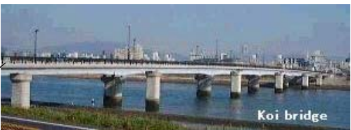
己斐橋 [水門+4140m/3080m+艇庫]
