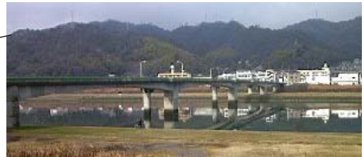
山手橋 [水門+3130m/4090m+艇庫]
